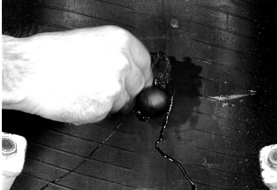
Applying vulcanizing cement to the buffed surface.
